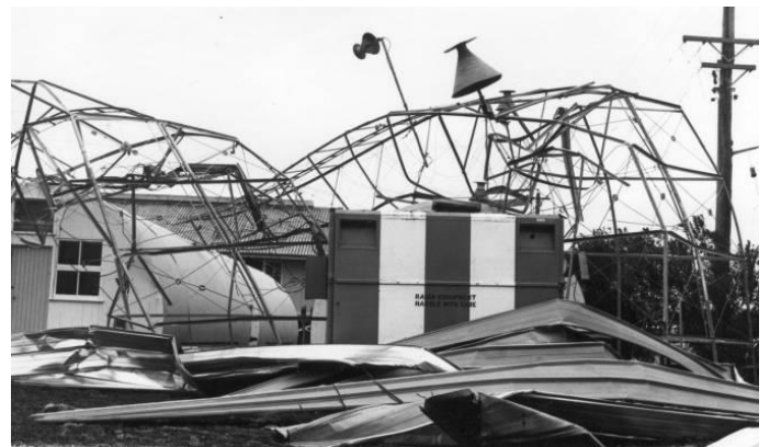
Damage to Radio Antennae Masts
